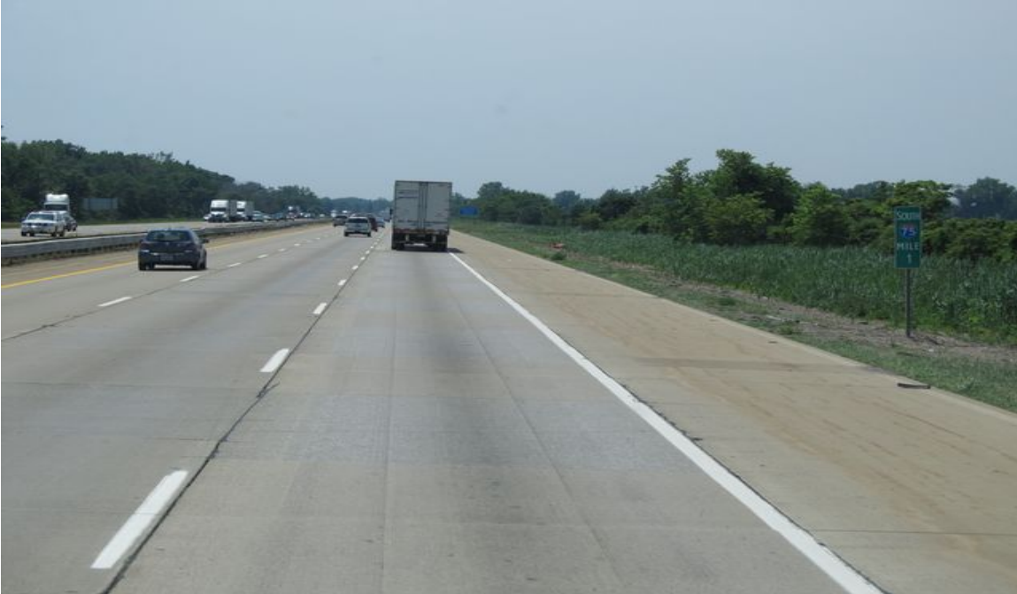
Figure 9: Measurement location 2: Interstate-75 Freeway with low traffic.
